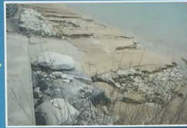
Beach Erosion caused by Stormwater Runoff →
