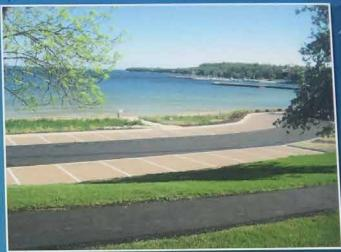
20 additional parking stalls were created, nearly doubling parking capacity. The project has been well received by the community. The permeable pavers are performing as expected and will continue to be monitored.
