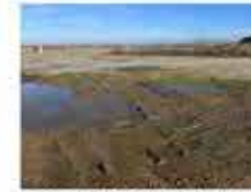
E. PONDING AT LOOKOUT - HEAVY VEHICULAR USE
