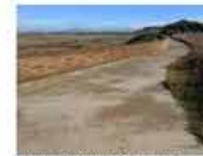
K. WALL DRAINAGE STRUCTURE - FUNCTIONING PROPERLY
