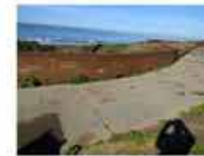
B. WALL DRAINAGE STRUCTURE - NO PONDING
